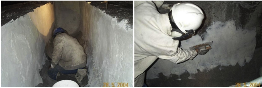
Fig. 14. Use of ceramic coating in CSN BF #3 Runners.
